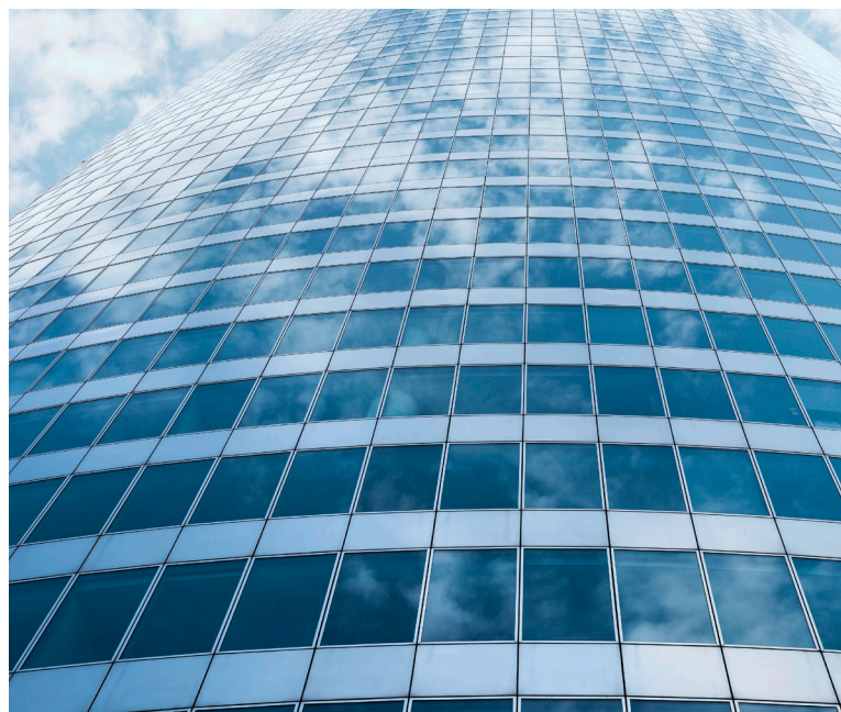
Krypton as filling gas for double-glazed windows
