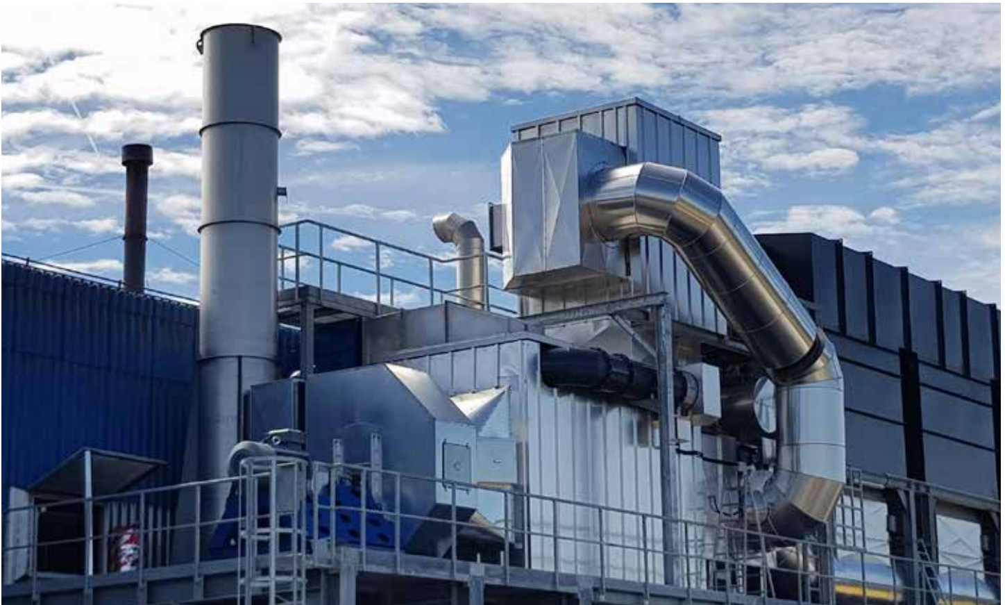
Regenerative thermal afterburning for cleaning of solvent-containing exhaust gases with integrated heat recovery for hot air and steam.
